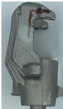
a) Claw corrosion
