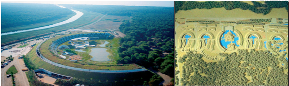
The resort Nuova Concordia, Italy (Arch. E. Ambasz) – example of “green architecture” ( http://ambasz.com/ /portfolio/specialized/Nuova-Concordia )
