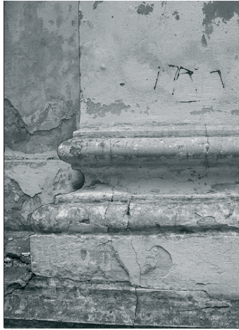
Fig. 2. The basis of pilaster made with using Roman cement. Foto: M.Bevz.
