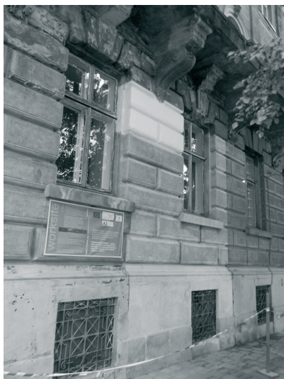
Fig. 4. The fragment of elevation of former “Palace of Justice” after the cleaning, made under promotion prof. J.Weber during the workshop in Lviv as the cooperation between the EU-FP7 project N226898 ROCARE. Aim was to demonstrate the possibility to recover the genuine appearance of the historic elevation by the use of Roman cement as historically authentic and compatible material. Executors were: Atelier Gurtner Wien (Austria) in cooperation with the restoration team of Department of Restoration of architectural Complexes of L'viv Polytechnic. August, 2011.
