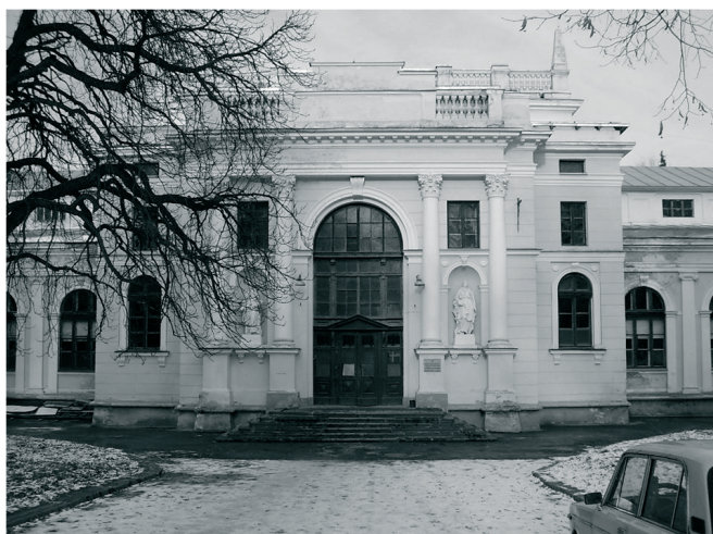
Fig. 1. The elevation of former Palace of Arts. Foto: M.Bevz, 2009.
