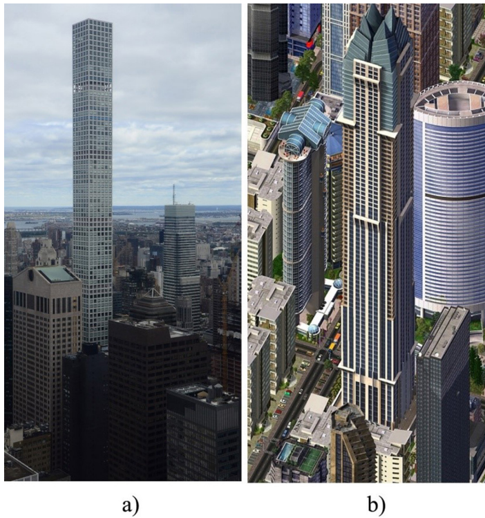
Fig. 4. Super-tall residential towers: a) 432 Park Avenue (New York, photograph by authors), b) Marina 101 (Dubai, developed by authors based on [28])
