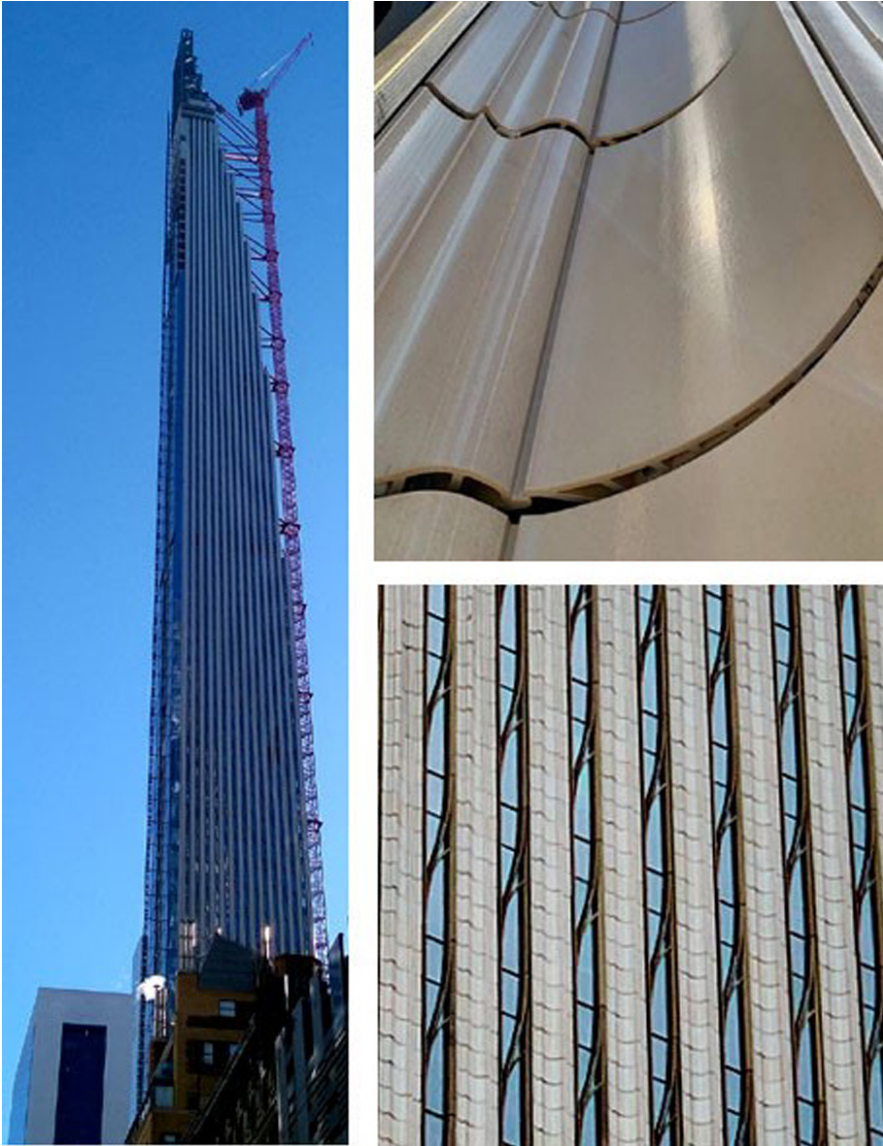
Fig. 10. 111 West 57 th Street (photograph by authors)
