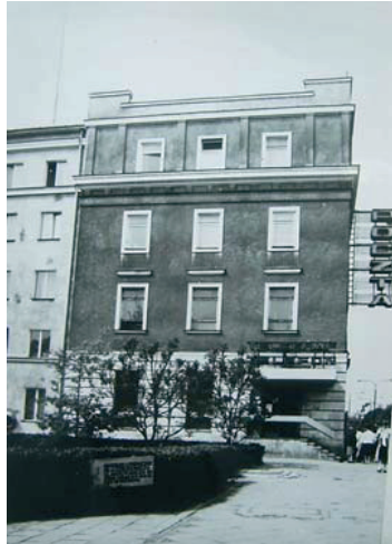
Photo 1. View of the Main Post Office Building after the repairs held in the 70 – ties.
