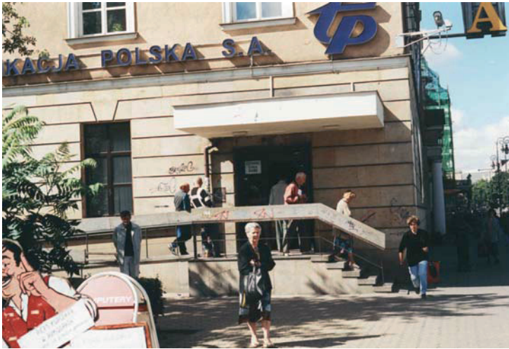
Photo 5. View of the entrance to the building in Czechowicz Square, 2001.
