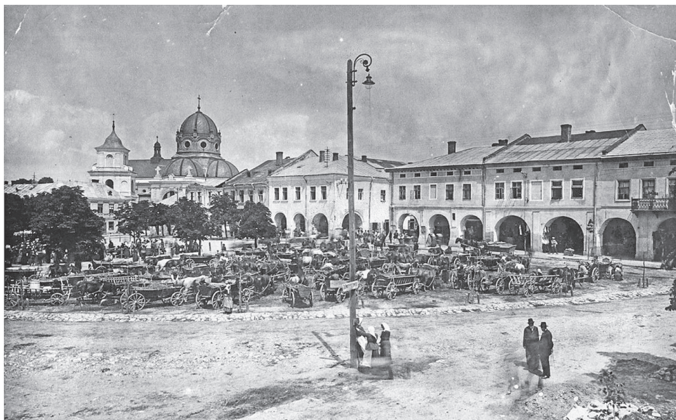
Fig. 2. Photo of central square of town of Zhovkva (Żółkiew) at the beginning of 20th century. The blocks of late Renaissance buildings with loggias-arcades in parter (northern part of square) ( http://www.polona.pl, zolkiew, 10.11.2018 ) [16]
