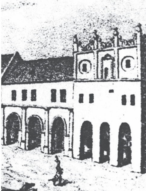
Fig. 6. Buildings with loggias-arcades in the central part of town of Zhovkva (drawing of beginning of the 19 th century) Zhovkva. Atlas ukrayinskykh istorychnykh mist. T. 3. Sc. Editor M. Kapral, Lviv, 2016, p. 32) [15]
