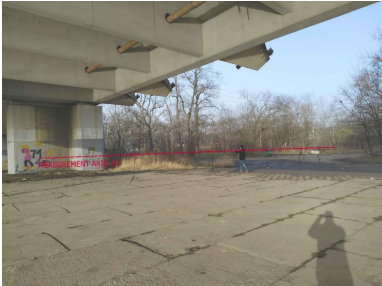
Fig. 16. Axis #3 was placed near the river bank on the area paved with concrete slabs (below the slope). Source: author's Piotr Kozłowski own photo archive
