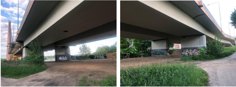
Fig. 9. Photos of the examined area. Milenijny Bridge (left-bank flyover) – crossing over the Odra River with access roads as part of the city-centre bypass, the section from Legnicka Street to Osobowicka Street, Wrocław – span № 7, between 7 th and 8 th axis – measurement axis #2. Source: author's Elżbieta Komarzyńska-Świeściak own photo archive
