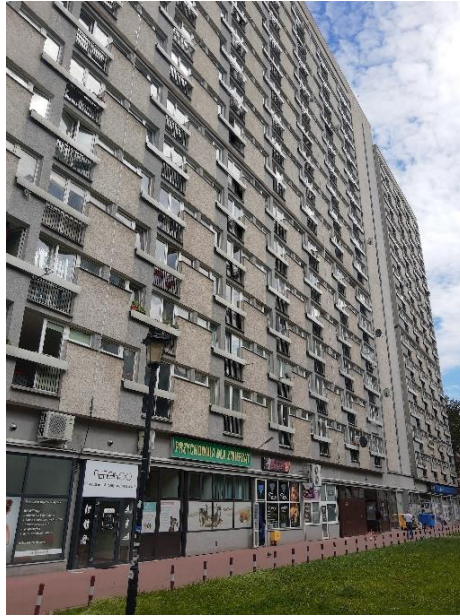
Fig. 1. The building from the estate „Za Żelazną Bramą” in Warsaw – the view. Source: Photo by the author
