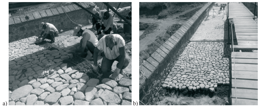
Fig. 8. a-b) The restoration of original flooring in accordance with its original
