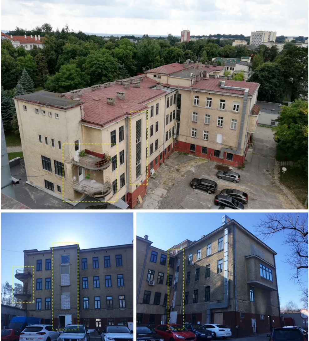
Fig. 9. Removal of glazing relevant to the modernistic form of the building in the process of its modernisation - loss of elements that characterise the building, routing of ventilation ducts along the elevation of the building, balconies to be demolished, lack of respect for the historic substance, Puławy, prepared by the authors, 2022
