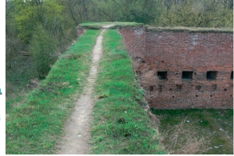
Fig. 29. Soft capping securing the castle wall crest. (The castle of Toruń-Dybbów)
