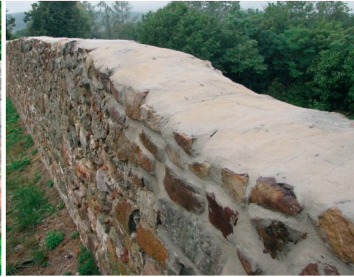
Fig. 27. The crest secured with a mortar layer – with molded inclination. (The castle in Bodzentyn)
