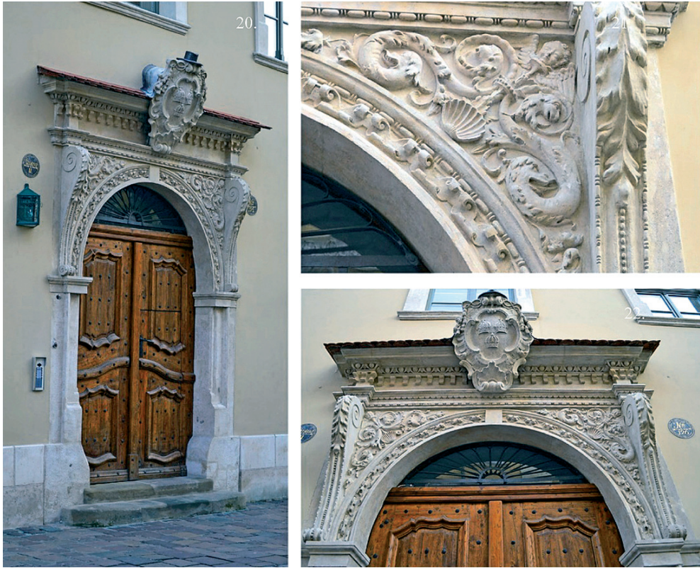
Lintel of a historic tenement house at 18 Kanonicza Street in Cracow
