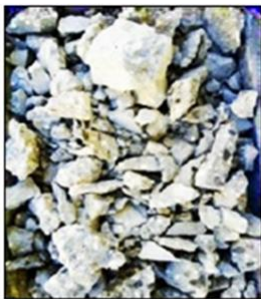
a) manual crushing of concrete slabs into smaller pieces
