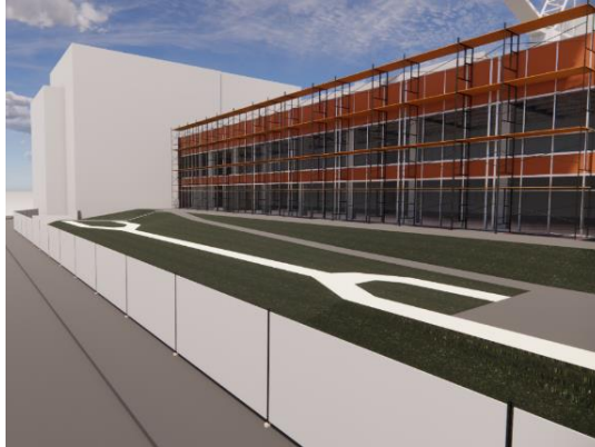
Fig. 2. Visualization of scaffolding for dismantling the front facade of the Tawo building, own elaboration
