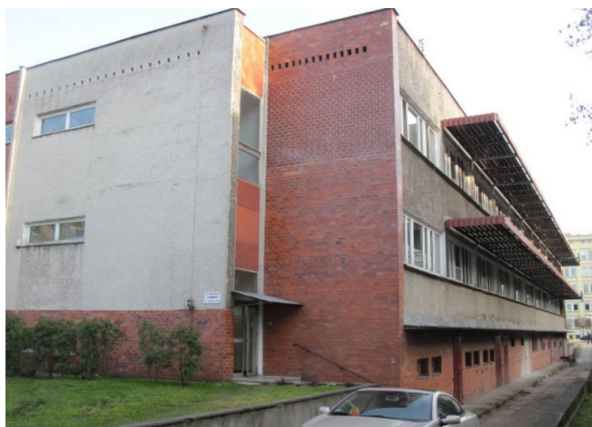
Fig. 7. Southern and western façades - 2009. Source: archival documentation of AGH
