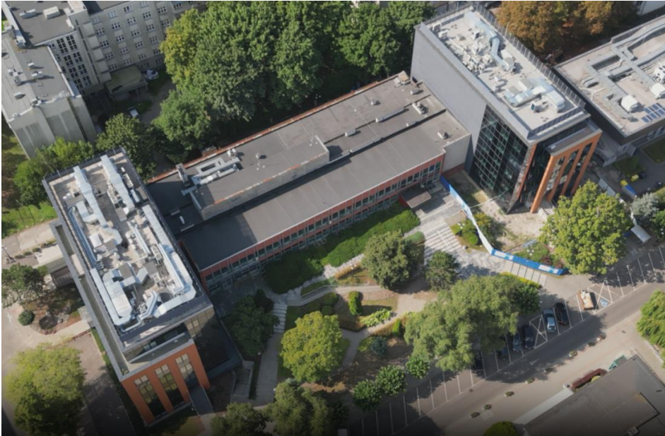
Fig. 12. Drone aerial survey – northern side, Source: private archive of the AGH Technical Department inspector, 26 August 2023
