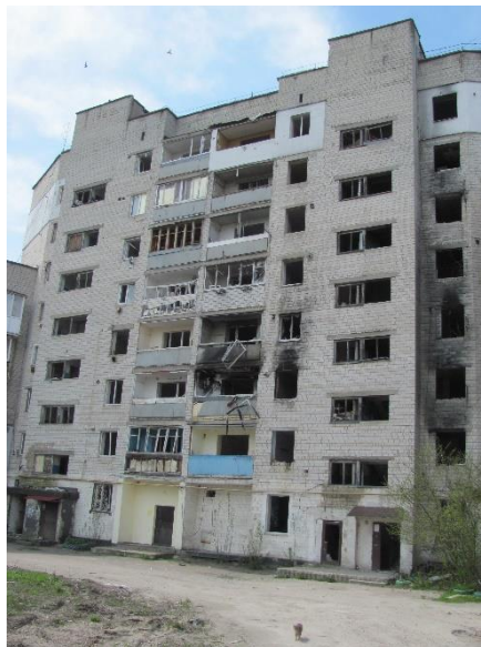
Fig. 2. Facade facing the yard along axis 'A'
