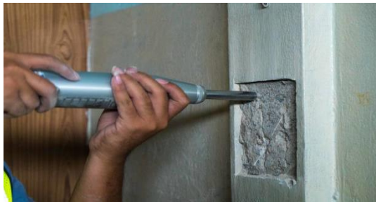
Fig. 5. Schmidt rebound hammer
