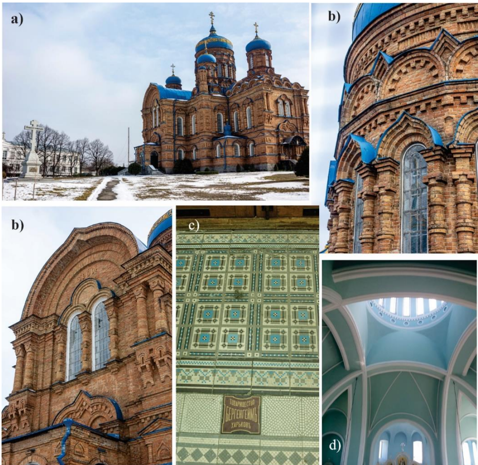
Fig. 4. The current state of the Cathedral of the Nativity of the Virgin: a) view of the cathedral from the northwest; b) brick decoration of the facade; c) authentic floor tiles; d) the construction of the intersection of four arches that supports the drum of the main dome, freeing the interior space from columns. Source: own study
