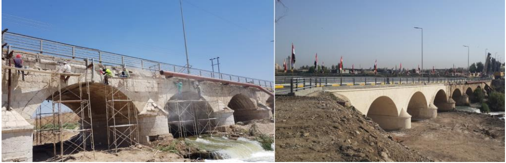
Fig. 6. Mosul Stone Bridge during the final stage of reconstruction. Source: [researchers]
