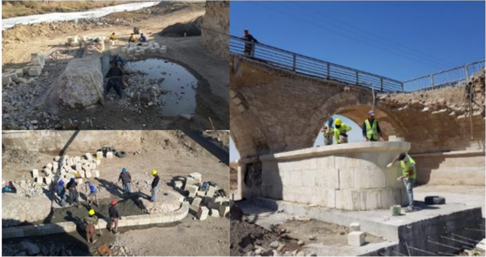
Fig. 4. Locating the destroyed pillar and rebuilding it. Source: [researchers]
