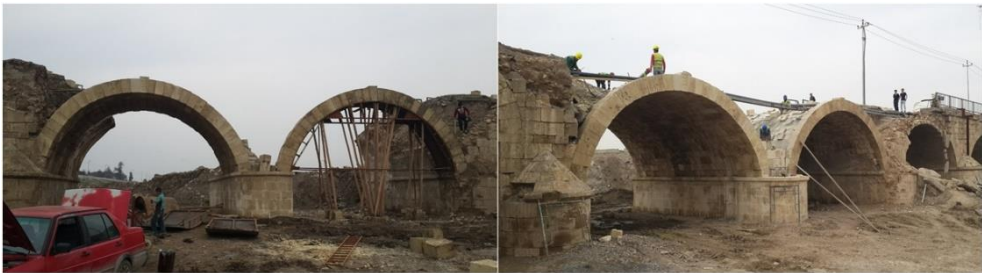
Fig. 5. Installing iron molds and constructing arches for destroyed vaults. Source: [researchers]
