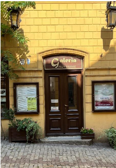
Fig. 4. Narrow entrance door leaf, step, and significant slope of the terrain in front of the entrance; Source: Author
