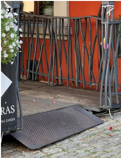
Fig. 7. A ramp instead of a step in the outdoor dining area; Source: Author
