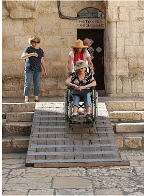
Fig. 1. A wooden ramp added to existing stairs in Jerusalem, providing wheelchair access to the Church of the Holy Sepulchre. Source: [19].
