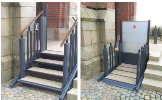
Fig. 9. Stair lift as an alternative to entrance stairs; Source: [25]
