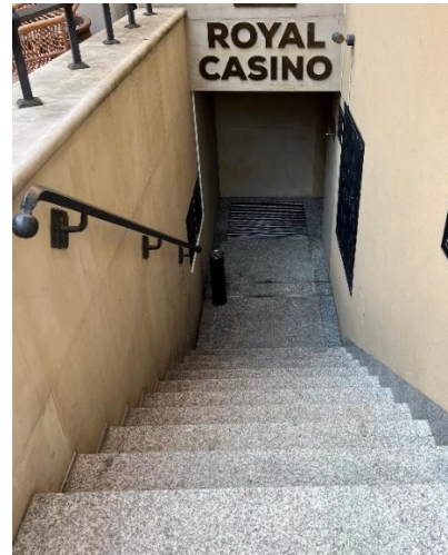
Fig. 8. Smooth stair surface with handrail; Source: Author
