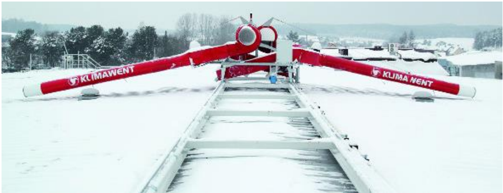
Fig. 15. Roof snow removal system based on materials from Klimawent S.A. company [16]
