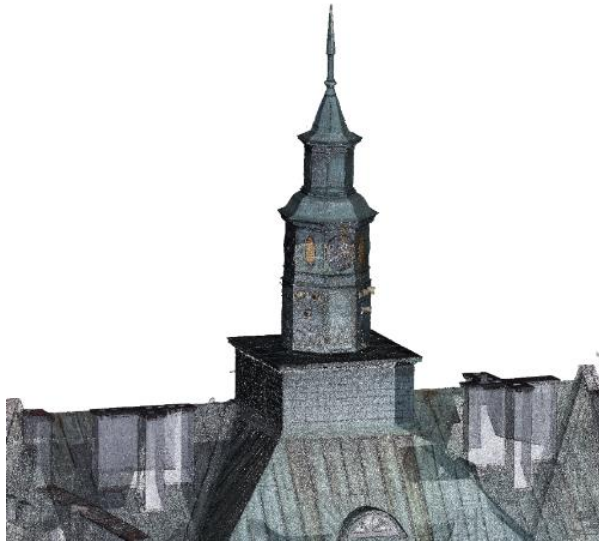
Fig. 6. Point cloud obtained through the photogrammetry method
