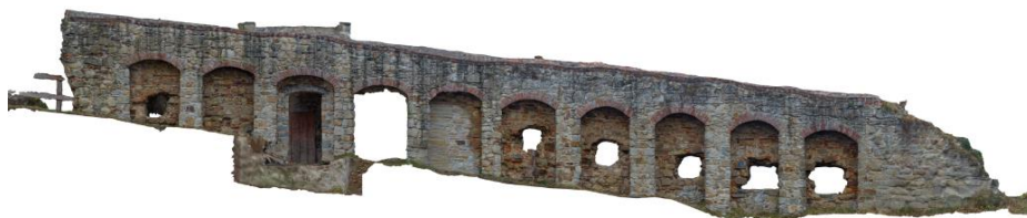
Fig. 15. Cross-section of the point cloud on the surface of the castle ruins
