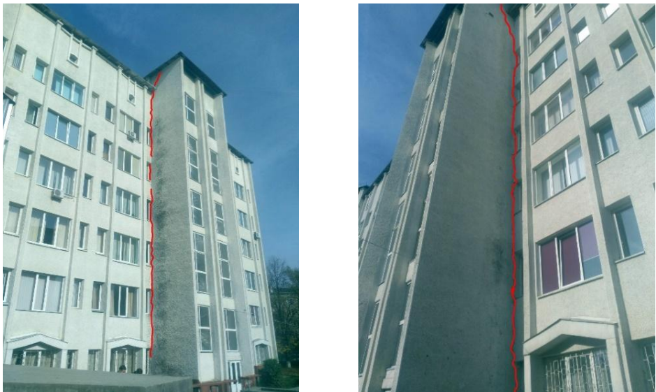
Fig. 4. Photo documentation of cracks No. 1 and No. 2 on the building facade. Source: the author's research
