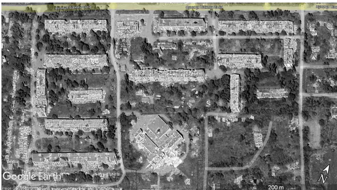
Fig. 8. Satellite image of the extent of destruction in a part of Popasna. Source: [21]
