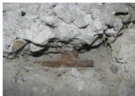
Fig. 11. Disclosure of the external wall at the intersection of axes "2"-"E" (general view of the longitudinal rod \varnothing 25 AII (A300C) and transverse reinforcement \varnothing 10 AII (A300C))
