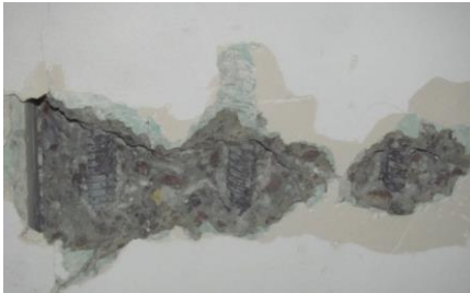
Fig. 13. Disclosure of a precast slab 1200 mm wide (a general view of three longitudinal rods Ø28 AIII (A400C))
