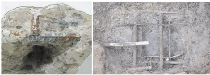
Fig. 17. Disclosure of the crossbar from the shelter room and mechanical opening of the monolithic section of the roof (extreme longitudinal reinforcement is Ø32 AIII (A400C), transverse reinforcement is Ø22 AIII (A400C))
