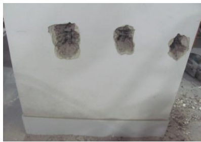
Fig. 9. Mechanical opening of column reinforcement at the intersection of axes "2"-"C"
