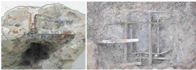
Fig. 17. Disclosure of the crossbar from the shelter room and mechanical opening of the monolithic section of the roof (extreme longitudinal reinforcement is Ø32 AIII (A400C), transverse reinforcement is Ø22 AIII (A400C))
