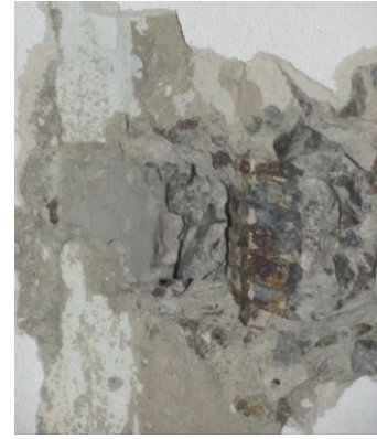
Fig. 15. Disclosure of a precast slab 800 mm wide
