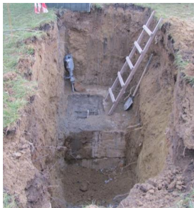
Fig. 6. The embankment removals above the shelter roof at the intersection of axes "2"- "E"
