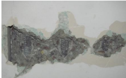
Fig. 13. Disclosure of a precast slab 1200 mm wide (a general view of three longitudinal rods Ø28 AIII (A400C))
