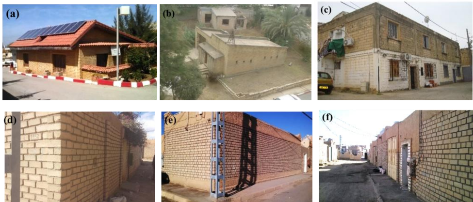
Fig. 1. Load bearing soil-cement blocks residential building in the a) Medenec prototype CNERIB-Algiers, b) Bioclimatic prototype CNERIB-Algiers c) Houses at Cheraga-Algiers, d) Tamanrasset building cities, e) Houses at Adrar, f) Houses at Moufflon – Tamanrasset
