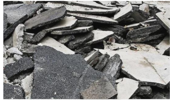
Fig. 1. Milling of existing asphalt pavements
