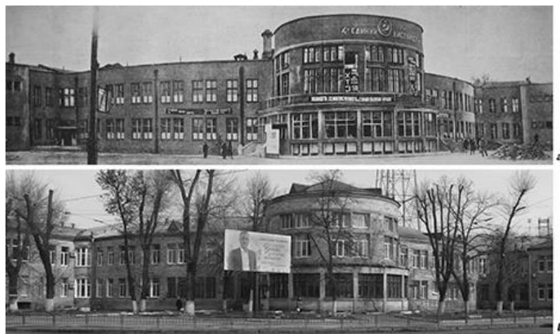
Fig. 6. Photographs of the 4th “unified dispensary”: a – after its construction in 1931, source: [35], and b – the current state of the building in 2013, source: own study
