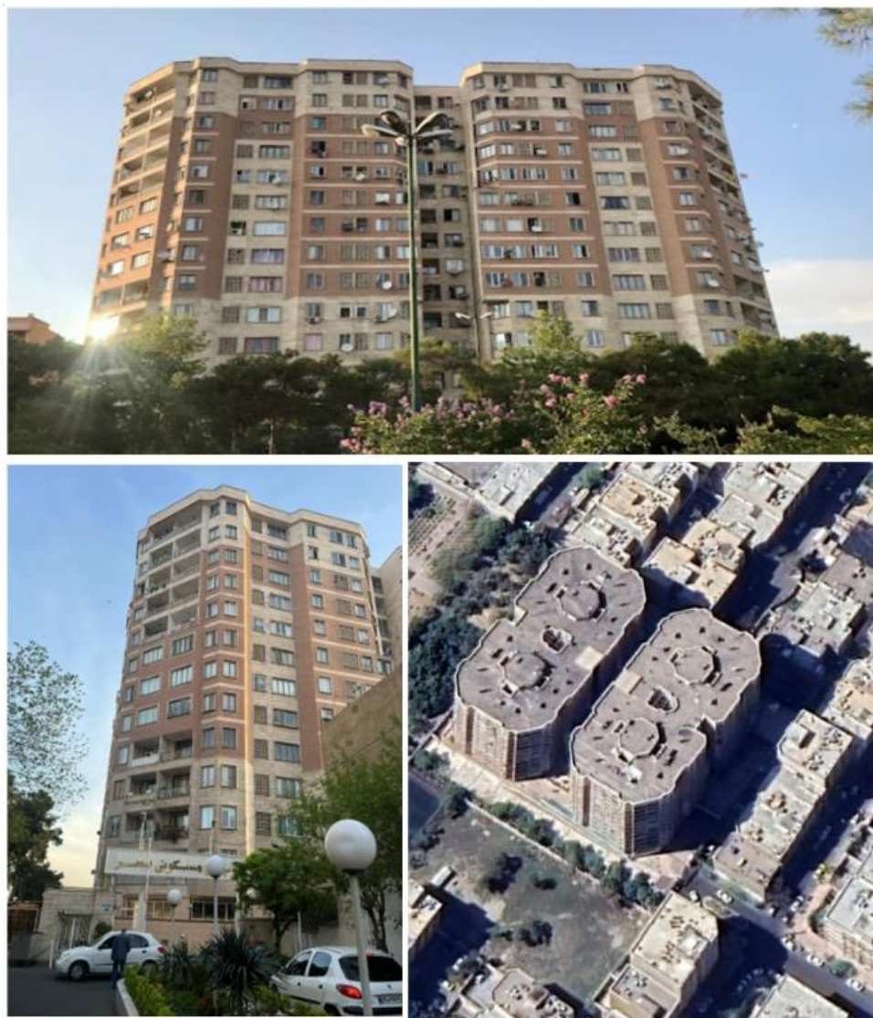
Fig. 3. Location of Sahar Residential Towers, its entrance view, and view from Shahrivand Park
