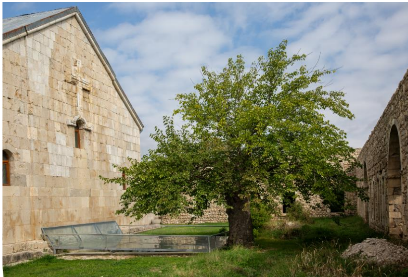
Fig. 3. The eastern facade of the church, photo by A. Balayan
