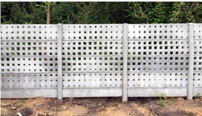
Fig. 5. The "Attractor" fence's realisation at the construction site. Source: [Marcin Giedrowicz]
