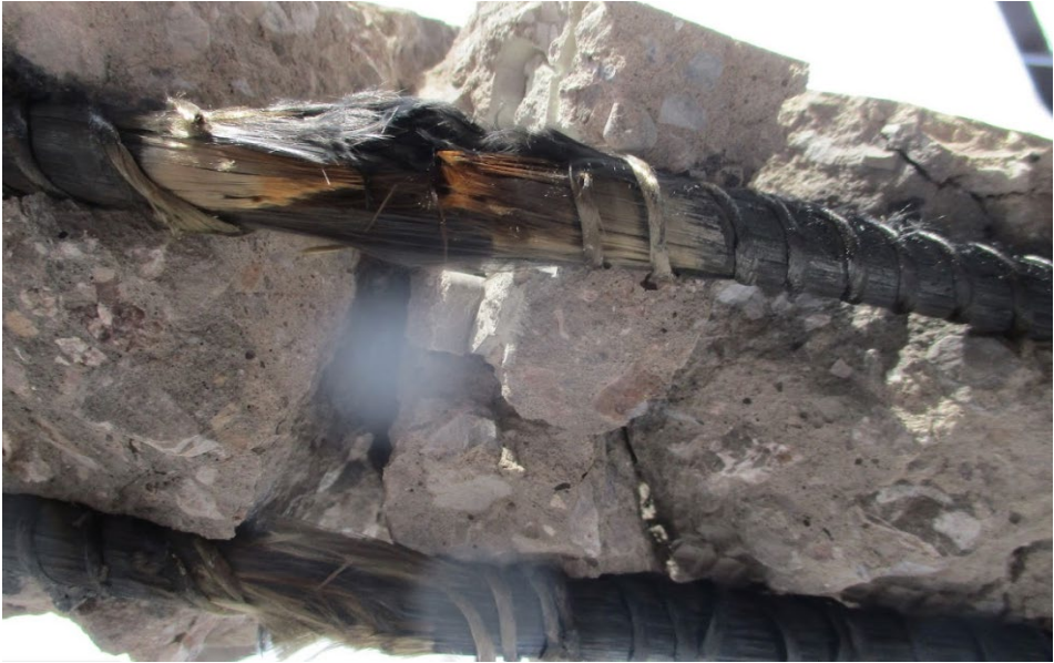
Fig. 4. Uncovered HFRP bars (by removing the clear cover after testing). Source: own study
