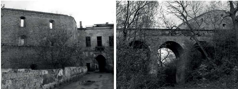
Fig. 2. Klevan Castle. Current status. View from the entry bridge. Photos by N. Leshchenko
