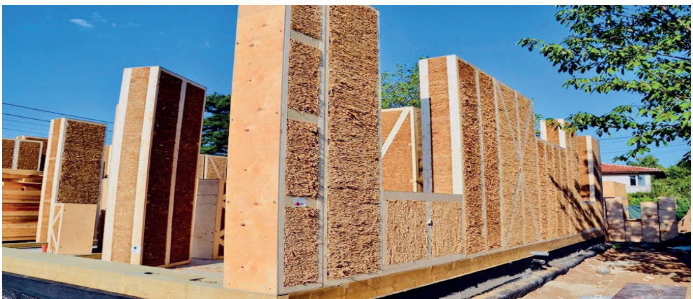
Fig. 3. Walls made of EcoCocon straw panels. Vastu Home – Bulgaria house design, source: www.ecococon.it
