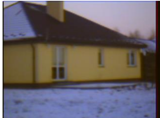
Fig. 7. View of the building under investigation
