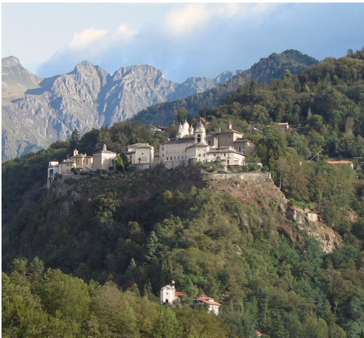
Fig. 1 View of the Sacro Monte di Varallo. Varallo is located in North-West Italy and in 2003, together with other eight Sacri Monti , has being recognized from UNESCO as a world heritage site
