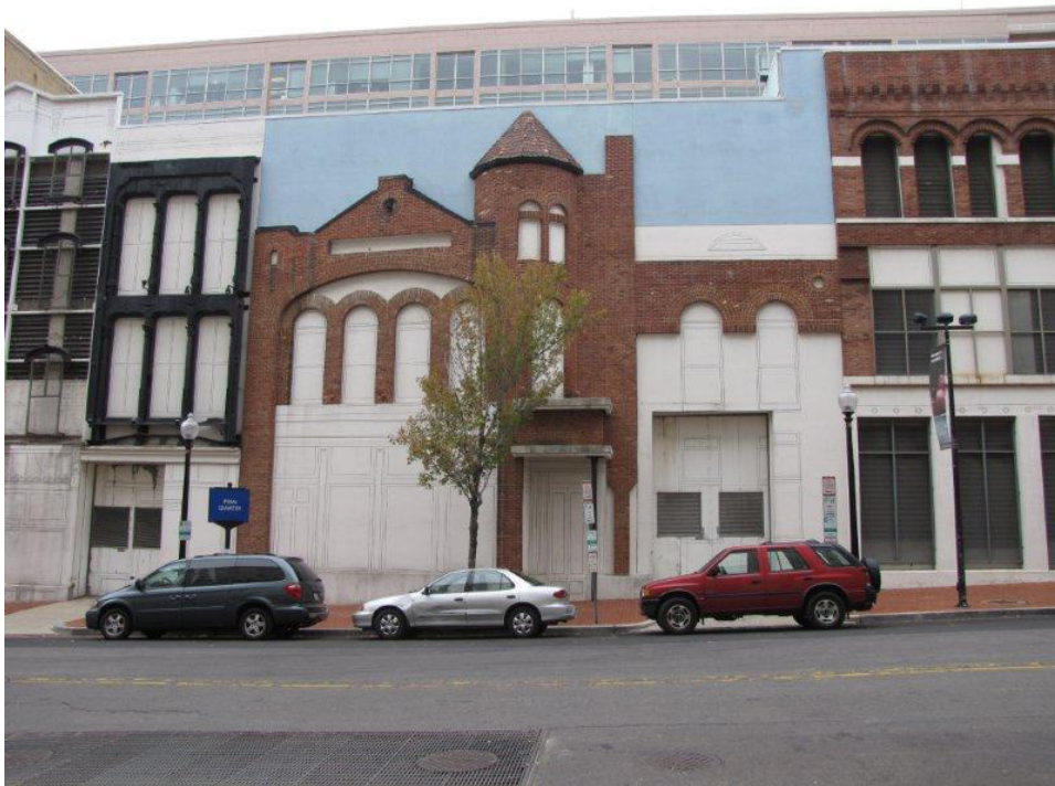
Fig. 1 Washington - the facades of historic buildings „glued” on the side wall of the shopping center; Photo: B. Szmygin
