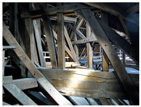
Fig. 1 Archival view of a fragment of wood truss structure in the transept of the Notre Dame cathedral in Paris, photo D. Mączyński 2009
