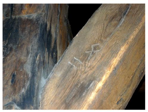
Fig. 3 Carpentry marking on an element of the roof truss of the Notre Dame cathedral, photo D. Mączyński 2009
