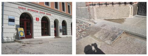
Fig. 3 A ramp incorporated into the surroundings of the historic building and a temporary ramp made of steel. (photo by the author)
