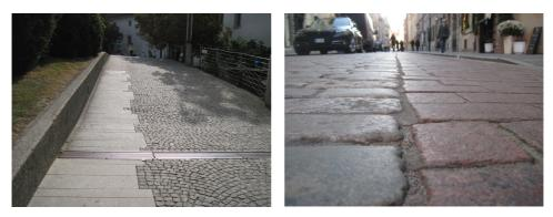
Fig. 2 An example of a surface of an access road leading to a historic object. Part of the surface is smooth or the smooth surface runs parallel to the rough surface (photo by the author)
