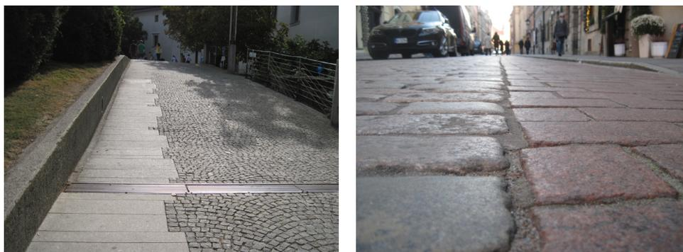
Fig. 2 An example of a surface of an access road leading to a historic object. Part of the surface is smooth or the smooth surface runs parallel to the rough surface (photo by the author)
