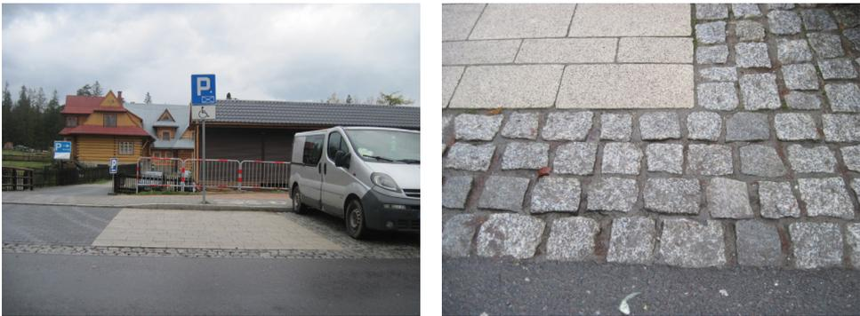
Fig. 1 An example of a parking lot with a split stone surface, where a smooth surface has been laid on the part intended for parking of a disabled person (author's photo)
