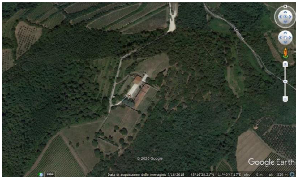
Fig. 2 Aerial view of the monumental complex of Villa Beatrice (© Google 2020)
