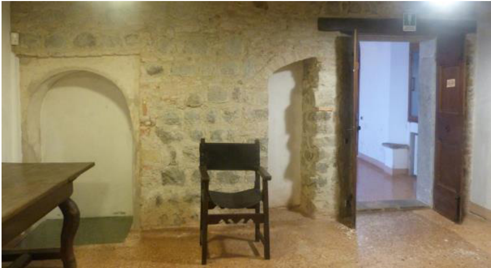
Fig. 10 Northern wall of Room B, where the remains of the ancient entrances to the medieval monastery refectory are visible. Below the floor level, it is a portion of the ancient medieval floor (on the left)
