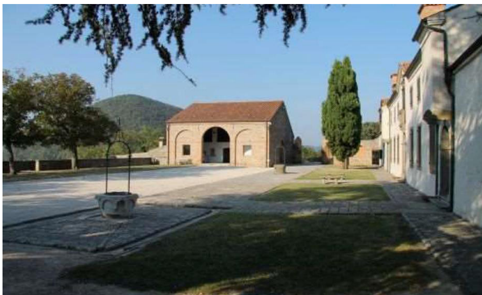
Fig. 5 The courtyard view from south with the modern barchessa and the two wells
