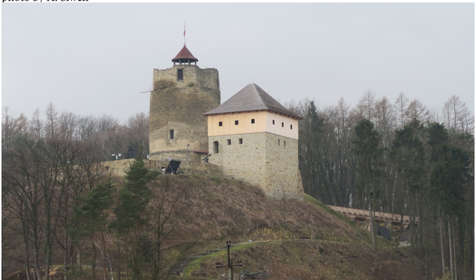
Fig. 4 Czchów - doubling of the castle's cubature as a result of reconstruction initiated by the local government, photo: A. Siwek
