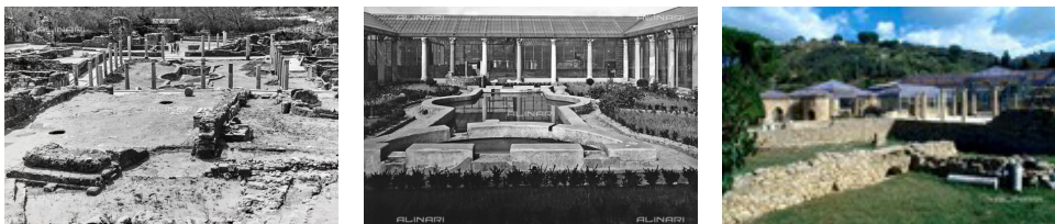
Fig. 9 Villa Romana del Casale in the years: 1954, 1962 and 90's, source: Alinari Archives, Firenze
