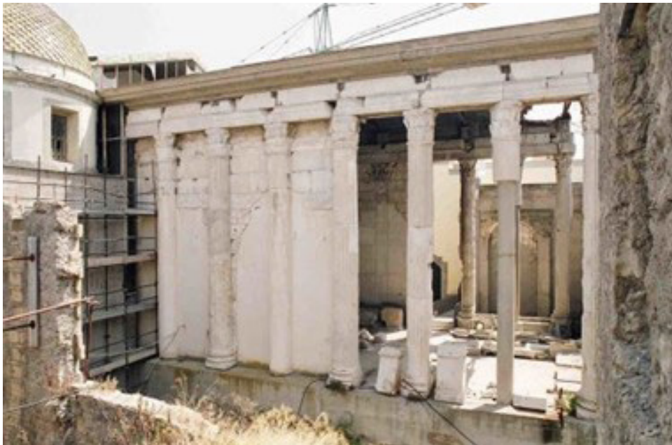
Fig. 12 Tempio Duomo Rione Terra before restoration work, source: http://1.bp.blogspot.com/-sq_JcdJgGbw/U5AVyZ0HuoI/AAAAAAAAAPRg/mTB15YaN5dM/s1600/fig.+2+--+Esterno+della+cattedrale+di+Pozzuoli.jpg
