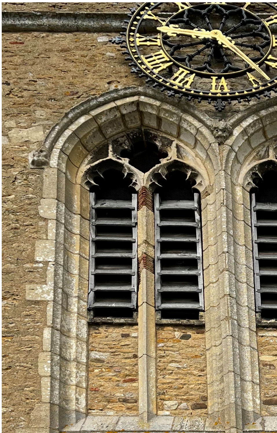
Fig. 2: The Parish Church of St Andrew, Swavesey – East Belfry Stonework
