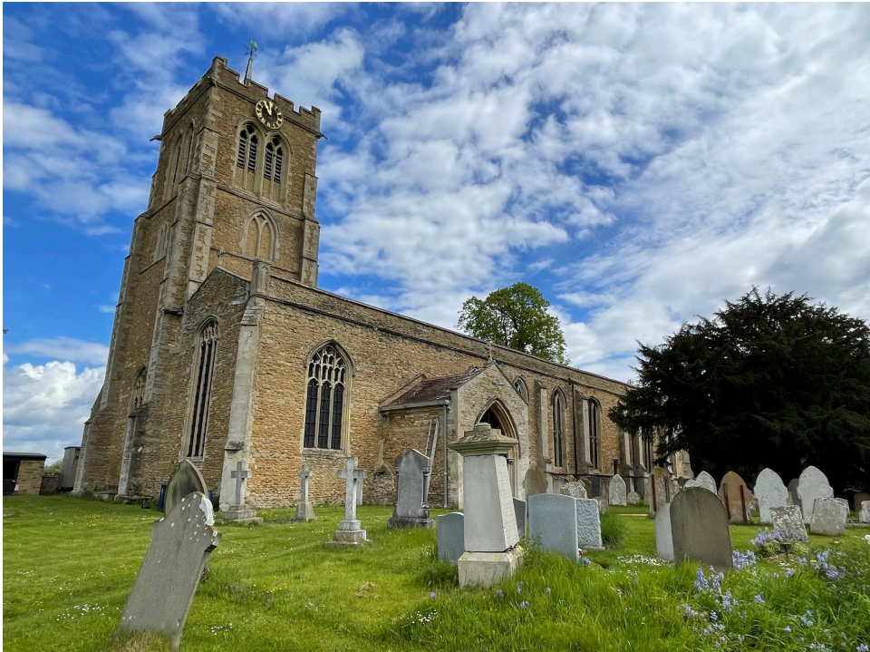
Fig. 1 The Parish Church of St Andrew, Swavesey
