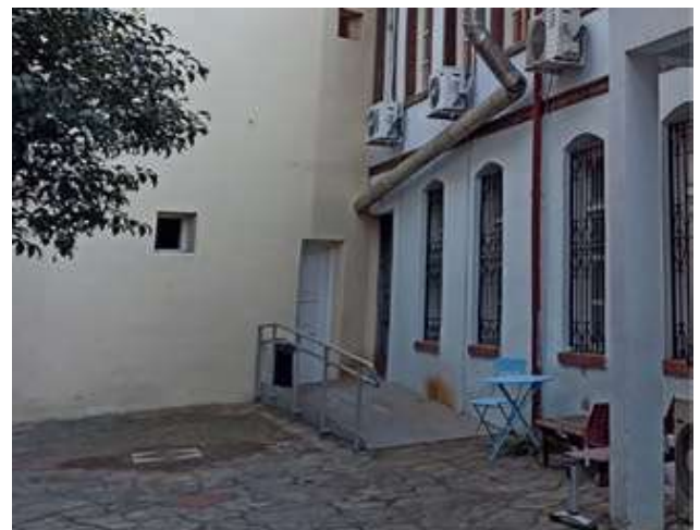
Fig. 11. Former residence in 25 Theophilou Street.
