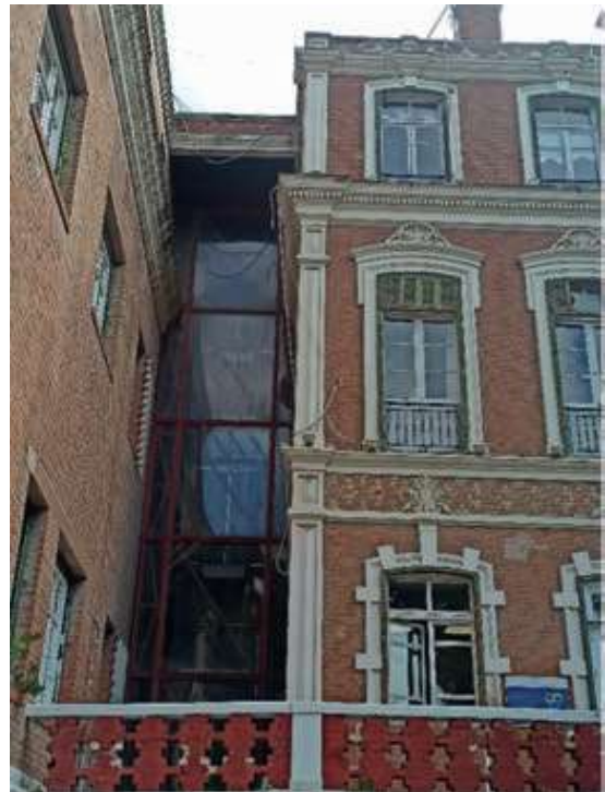
Fig. 15. The former Allatini Mansion.
