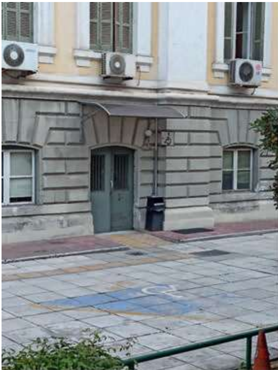
Fig. 12. Former Administration Building.
