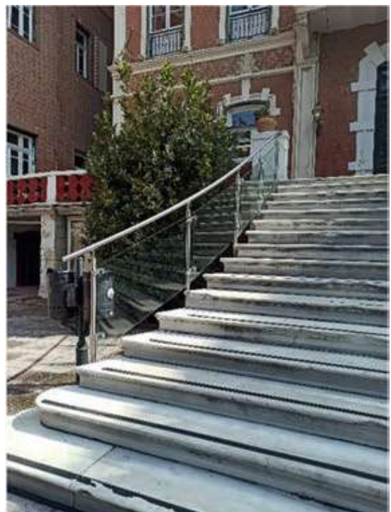
Fig. 9. The former Allatini Mansion.
