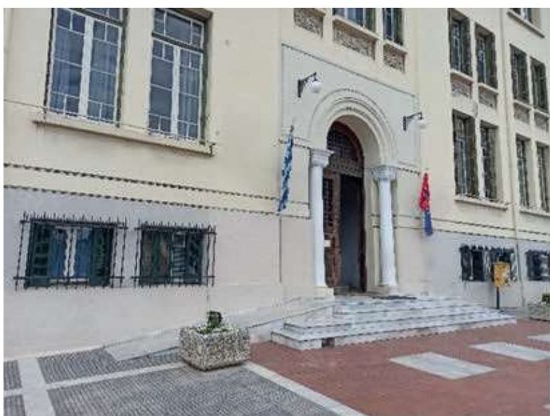
Fig. 4. The YMCA Building.
