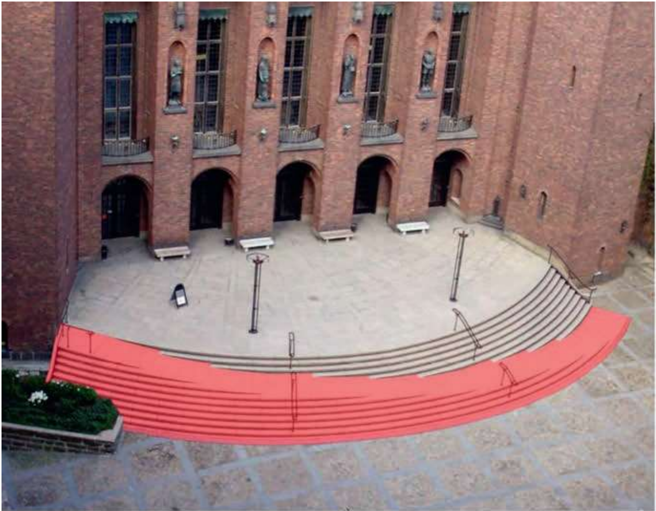
Fig. 5. Stockholm (Sweden), Wrangel Palace. The project retains the radial stairway and original materials, while adopting a solution that improves accessibility for people with disabilities.
