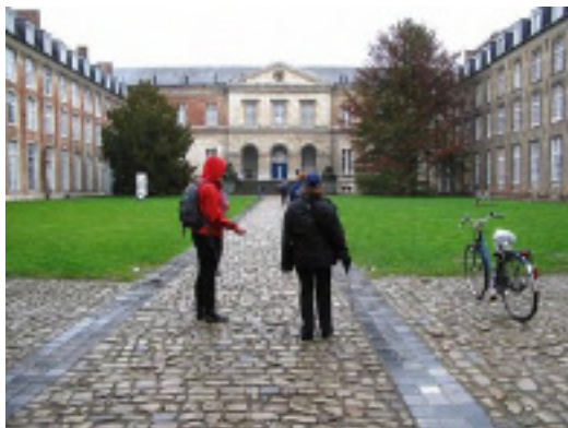
Fig. 5 A blind person uses the strip in natural stone as a guideline (© Van Bokstal)
