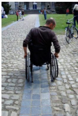
Fig. 4 A wheelchair user can not use the strip in natural stone as a comfort strip as it is too narrow (© Deraeve and Janssens)
