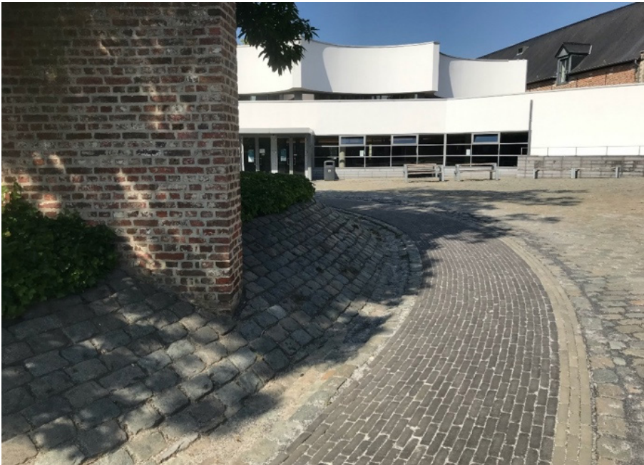
Fig. 9 Detail of the connection between the cobblestone pavement, comfort zone and central plant bed after the interventions. The right side of the new comfort zone is marked with a guiding line of brick pavers with a contrasting, lighter color. On the left, the edge of the path is marked with a roll layer in cobblestones. (© Van de Bemdt 2020)
