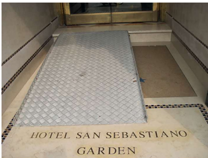
Fig. 12. Access to the building entrance with a ramp (without handrails) with a solid, corrugated running surface; Venice, Italy (photo by K. Kaperczak).
