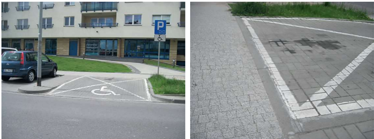
Fig. 8. Parking spaces made at the level of the adjacent sidewalk do not require overcoming height differences (faults) when accessing vehicles; Warsaw, Poland (photo by K. Kaperczak).
