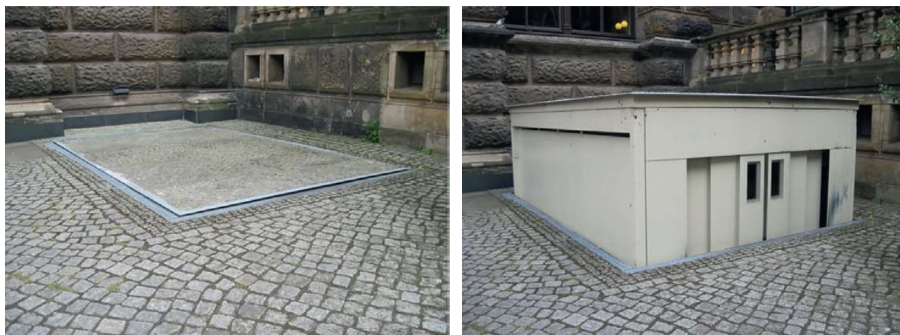
Fig. 16. Underground passenger lift, which takes the disabled person to an underground corridor; Zwinger Palace, Dresden, Germany (photo by K. Kaperczak).
