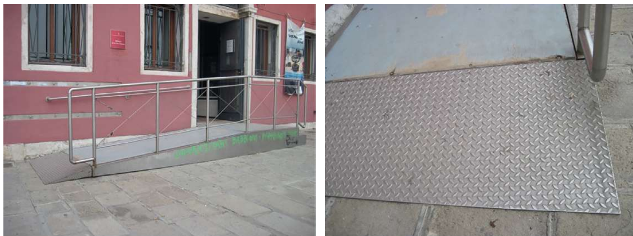
Fig. 13. Access to the building entrance with a ramp (with handrails) with a solid, corrugated and smooth running surface; Venice, Italy (photo by K. Kaperczak).
