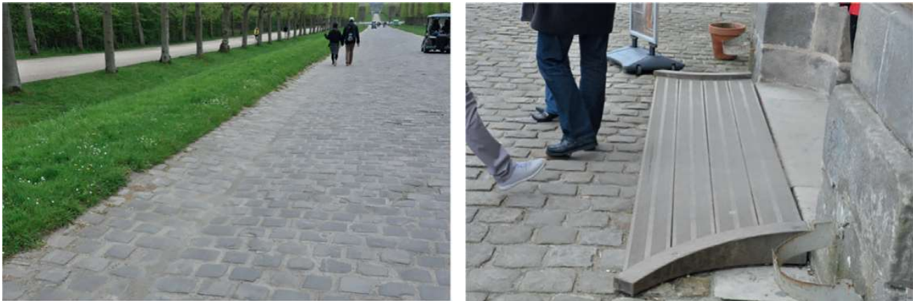
Fig. 3. The Grande Allée with stone paving and the Contre Allée with more comfortable mineral paving (left). Photo by D. Sikora, 2018. Wooden platform levelling the threshold at one of the entrances to the Palace of Versailles (right). Photo by D. Sikora, 2018.
