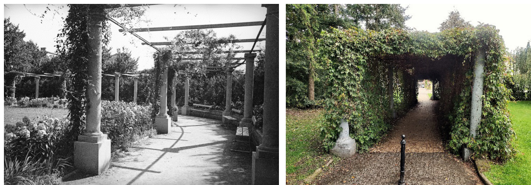
Fig. 34 Pergola at Hellwig's Parterres, 1930s and today. As a result of complete overgrowth with Parthenocissus , there are no links from the interior of the pergola to the area of the Parterres. Source: photo by H. Poddębski, ca. 1939, NAC, Unit Archiwum fotograficzne Henryka Poddębskiego, ref. 3/131/0/-/53/32; photo by M. Lisowska, 2022.
