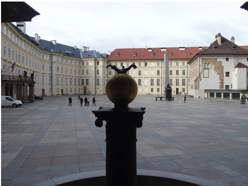
Fig. 6 Prague Castle. Third Courtyard, renovated 1926–1932, photo by the author, 2022
